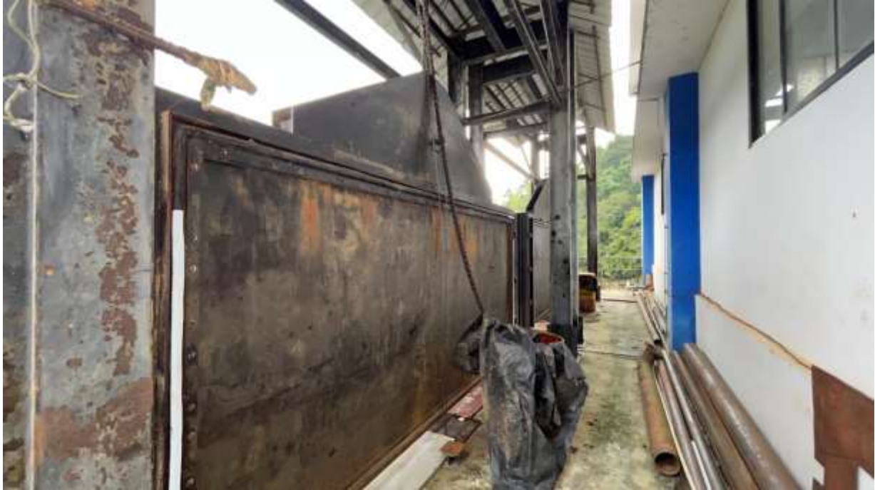
Fig 2.4 Draft tube Gate
