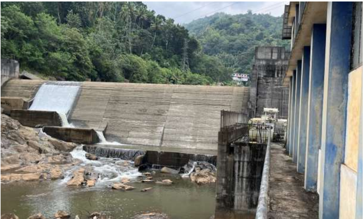
Fig 1.4: Photograph of Diversion Weir
