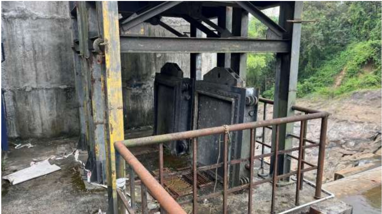
Fig 2.2 Closing arrangements of the Scour Gate
