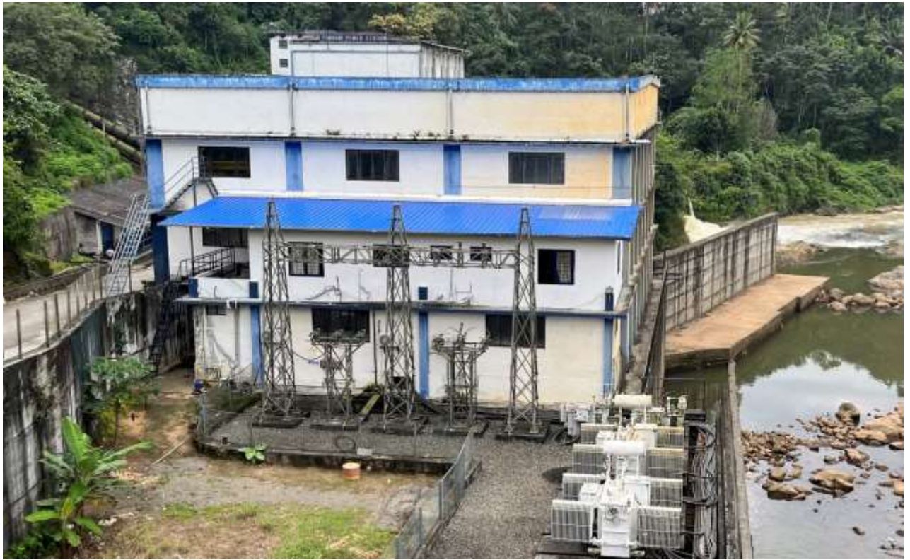
Fig 1.6: Power House – Vellathooval SHEP
